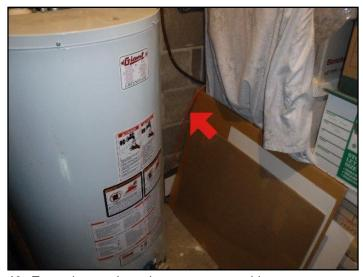
46. Extension cord used as permanent wiring
