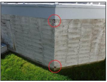
39. Parging damaged or missing
