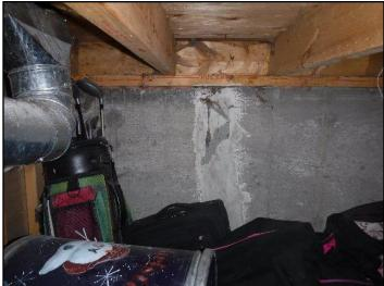
**35.** Typical minor cracks
