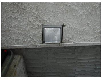
24. Caulking missing or deteriorated
