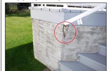
38. Parging damaged or missing
