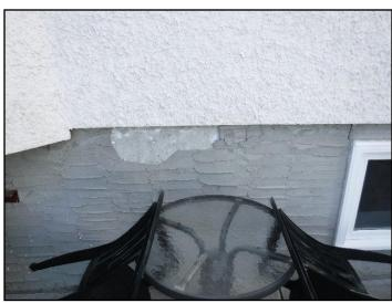
37. Parging damaged or missing
